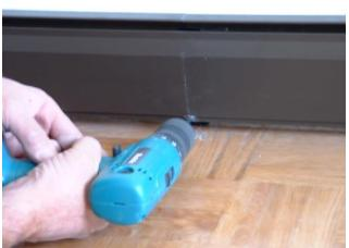
For wall longer than 2.5 m clip a complete lenght of skirting unit on the upper clip of the bracket and with a slight pressure from top to bottom.
