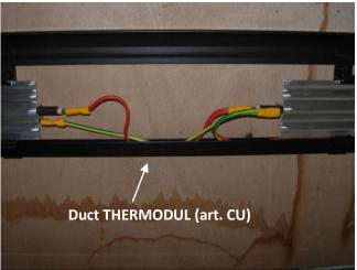
For the passage of cable, use art. CU of Thermodul,duct in aluminium for the passage maximum of 3 cable on 2.5 mm<sup>2</sup> to put with a slight pressure on the feet of bracket with the striped side on the wall (alternative it's possible use a pvc duct, the maximum size is 12 mm height and 7 mm width).
