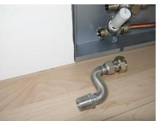
Encase completely the metal panel box on the wall, making sure that it does not stick out from the plaster, this could cause problems during installation (space). Protect the valve during plastering. Connect the piping arrangement.
