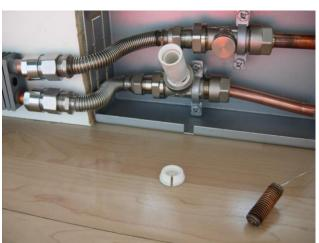
connect with the fitting 15-1/2F, directly between the flexible hose and the heating core.
