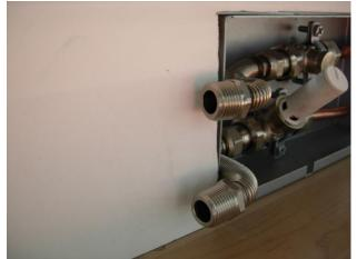
Repeat the operation for the holder. Bring the attacks at the same height Set the flexible hoses to the wall (as close as possible) so that it does not protrude more than they should. If they would that may cause problems in fixing the mask.
