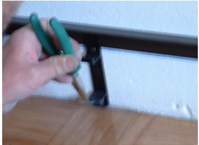
Before installing the skirting unit, ensure that the brackets are all at the same height.
