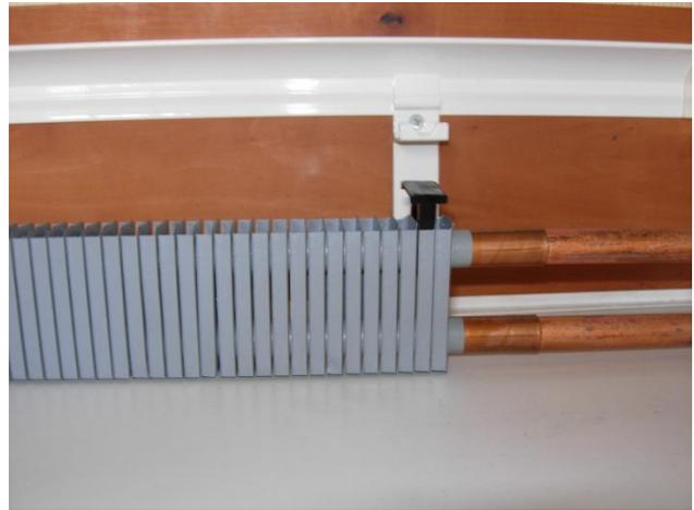
Before fixing the heating core (art. KA) and realizing the connections (welding ), place it on the wall and mark with a pencil the thin plate that will fall in the middle of the bracket (art. OT). If it is impossible to do this, measure the actual distance between the various brackets.
