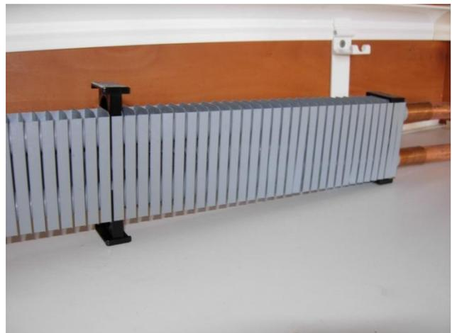
Once you have fixed the 2 clips repeat the operation on all brackets where the heating core is located. Place a pair of clips between the two brackets
