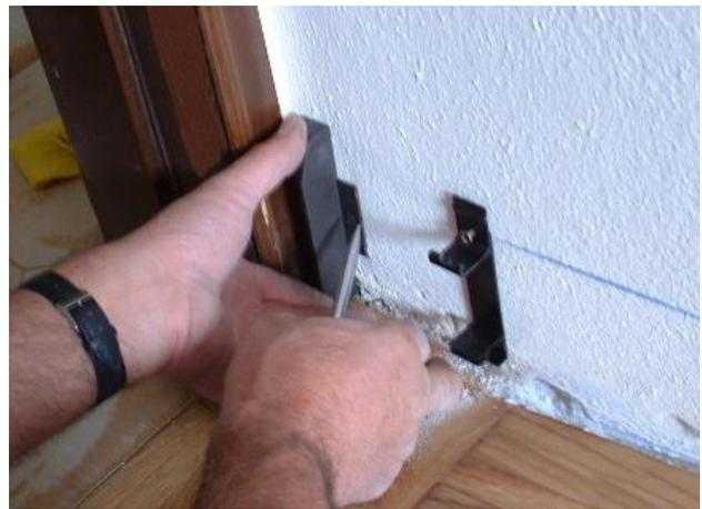
Screw the brackets tightly to the fix the upper profile to the wall
